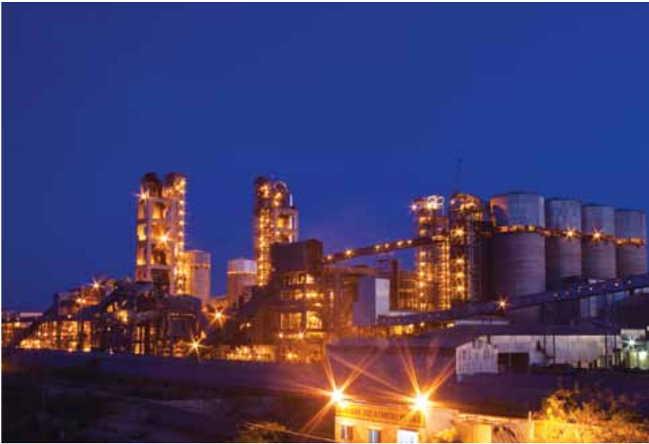
A view of Ariyalur Plant.
