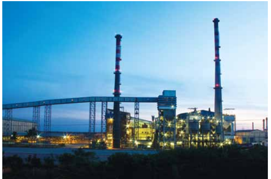
A view of Thermal Power Plant at Ariyalur.
