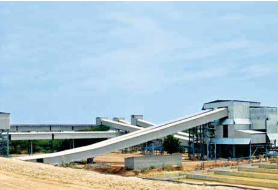
Limestone Benefication Plant at Alathiyur, commissioned during the year.
