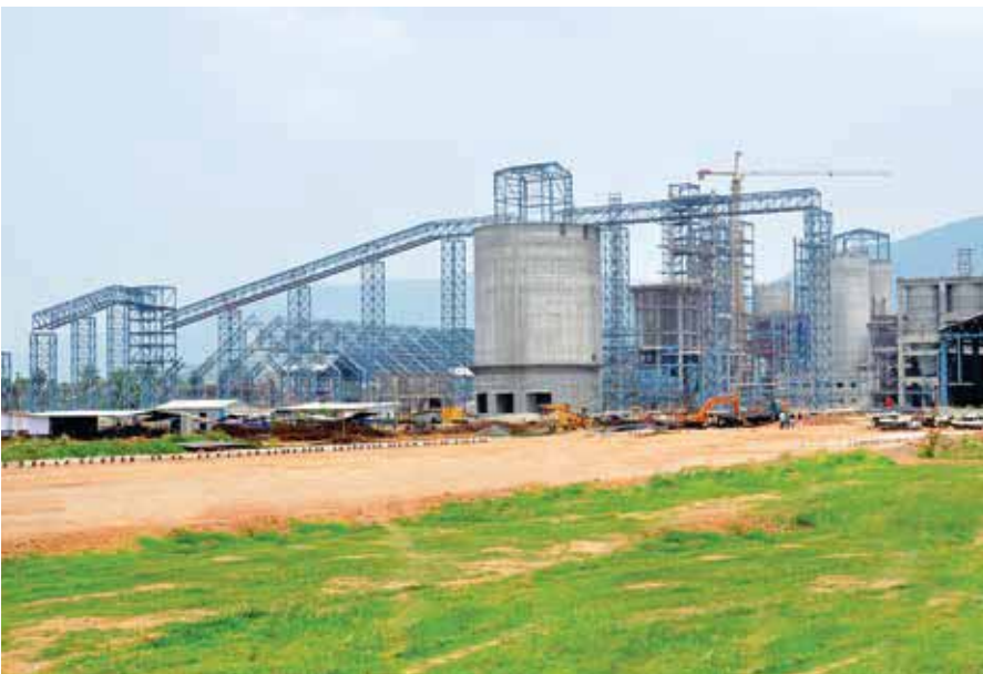
A view of Vizag Grinding Unit under construction.
